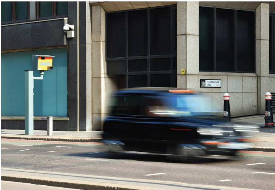
▼ Figure 7.1 Safety camera with sub-pillar
