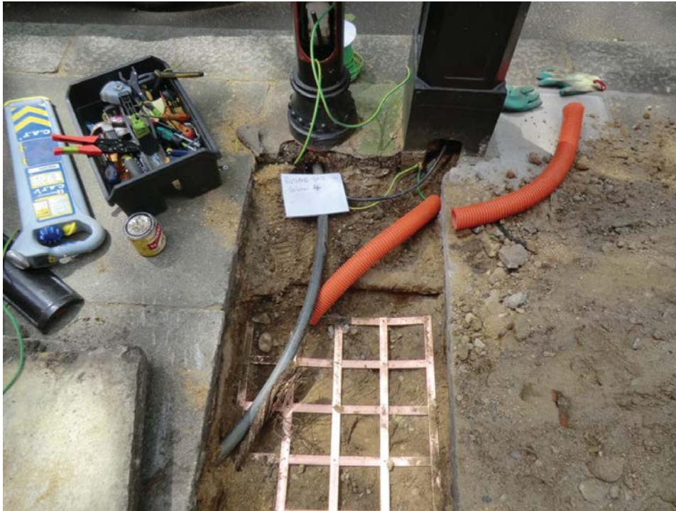
▼ Figure 2.3 Earth mat installations
