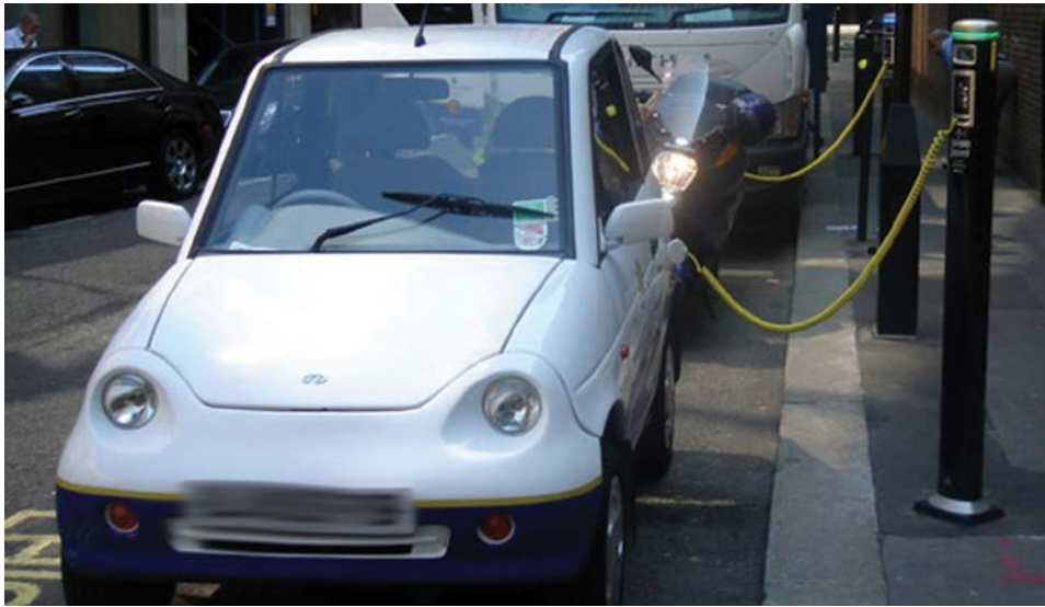
▼ Figure 5.2 Individual charge points and twin charge point with impact protection
