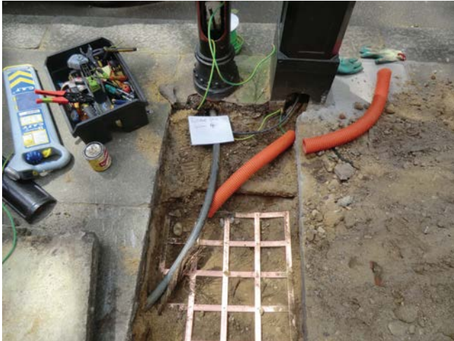
▼ Figure 6.4 Typical earth mat installation
