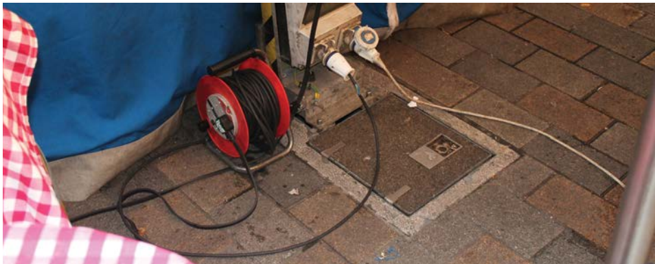
▼ Figure 6.10 Long extension lead that presents a trip hazard and a coiled extension lead presents a potential fire hazard
